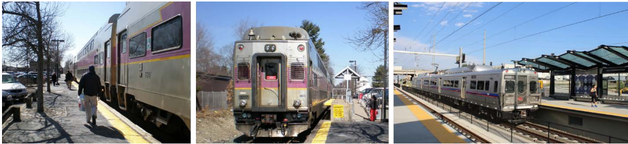
Left to Right: Low-Level Platform, Mini-High Platform, High-Level Platform
