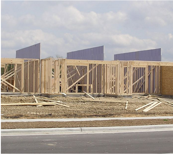
Wood frame fire separation walls
