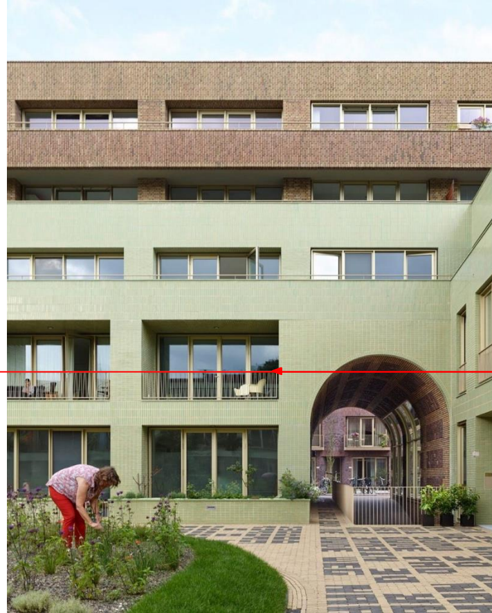
Multi story Unit
