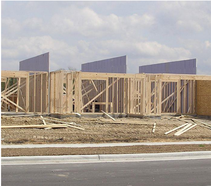
Wood frame fire separation walls
